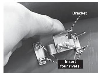
7. Using a rivet gun, fully install the rivets.
