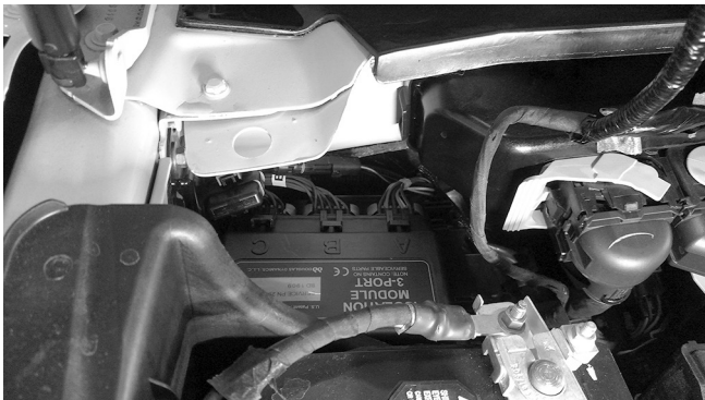
Isolation module, after installation.
